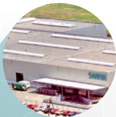
SANHA production and logistics center in Legnica, Poland
